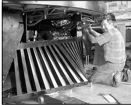
Darrell Arndt works on the installation of the new pilot for D&IM No. 25.
